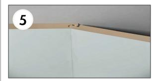
Starting at approximately 45°, angle the tongue of the next panel into the groove of the fixed panel. Ensure the tongue is fully inserted into the groove before snapping it back to the wall, otherwise it may damage the joint.
